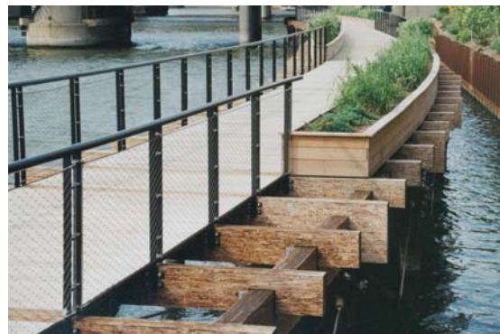
Cantilever deck (8’ width, with metal railings and metal supports) $300 per linear foot
