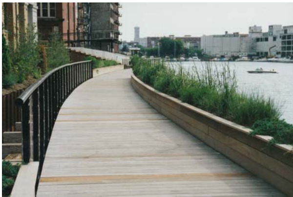
Wood boardwalk (8' width, includes wood railing and metal supports) $180 per linear foot
