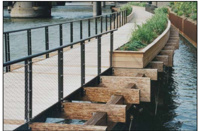
Piered segments should be explored with DNR for shallow riverfront lots – particularly on the west bank just above and below Milwaukee Street.
