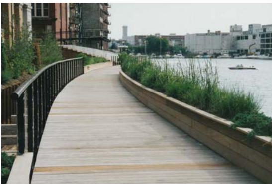
Wood boardwalk (8’ width, includes wood railing and metal supports) $180 per linear foot
