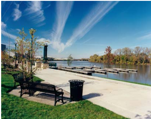
Concrete Pathway (8’ width, includes grading and plantings along edge) $54 per linear foot
